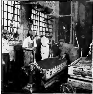
Fig. 60. Butting Off the Cope Half of Mould.
